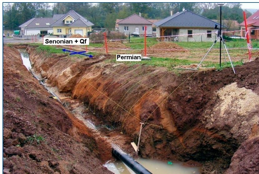
Fig. 2: View of the western end of the water pipe excavation south of the village of Úsilné. The contact between the Senonian sediments of the Budějovice Basin and the Permian sediments of the Lhotice Basin was uncovered by the trench. Senonian sediments and contact are covered by a layer of fluvial sands and slope sediments affected by gelifluction. Photo I. Prachař, 2009.
