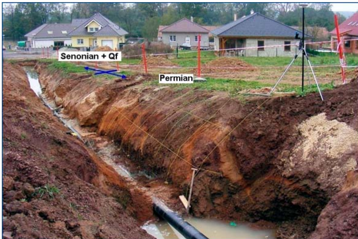
Fig. 7: View of the western end of the water pipe excavation south of the village of Úsilné. The contact between the Senonian sediments of the Budějovice Basin and the Permian sediments of the Lhotice Basin was uncovered by the trench. Senonian sediments and contact are covered by a layer of fluvial sands and slope sediments affected by gelifluction. Photo I. Prachař, 2009.
